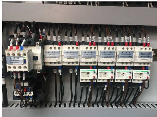
Schneider AC contactors
